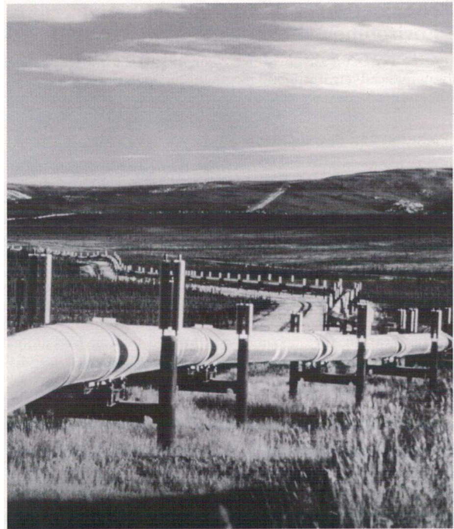
The Trans Alaska Pipeline
